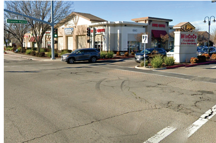
Retail building immediately west of the site
