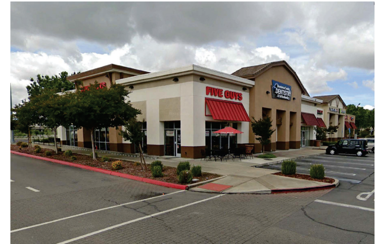
Retail building immediately west of the site
