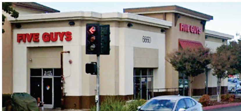
Copy from this adjacent example Projecting wall caps and brackets Recessed windows
