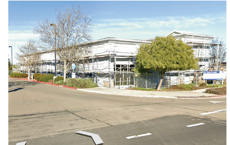
Retail building immediately east of the site
