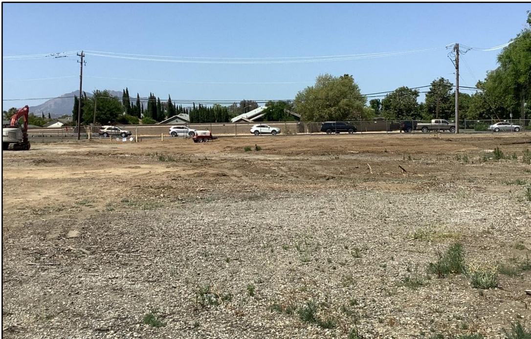
After building demolition
