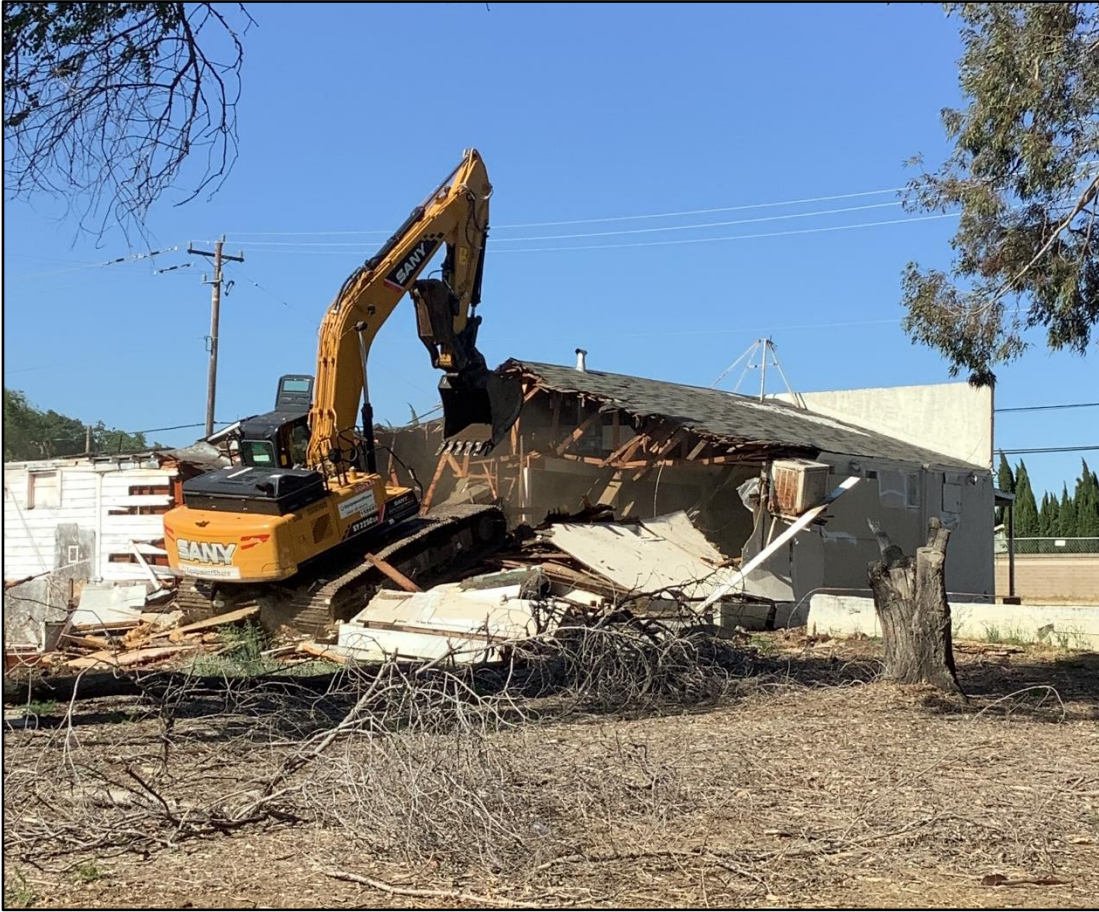
During building demolition
