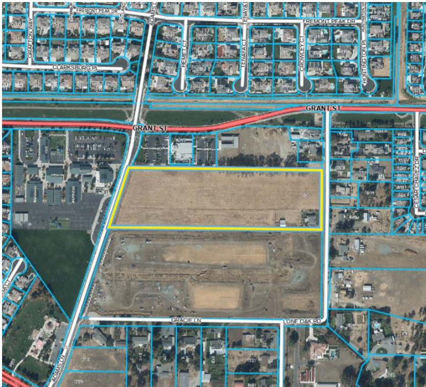
2023 Aerial Photo of Project Site
