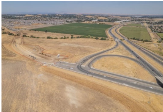
Sand Creek Road Extension
